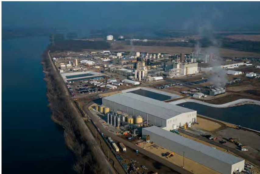
< 3M's Cordova chemical plant on the Mississippi River
