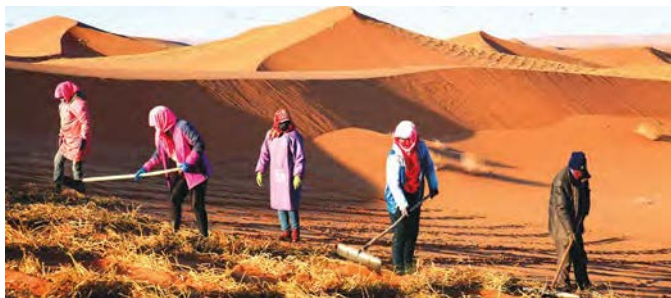
Sand control workers help prepare barriers that will house sand-resistant plants in Gansu province. YANG YONGWEI / FOR CHINA DAILY
